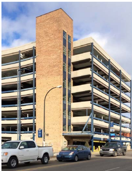
S.W. stair/elevator tower, before
