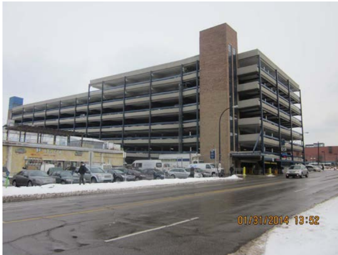
Fourth & William parking structure seen from Main Street, existing stair/elevator tower
